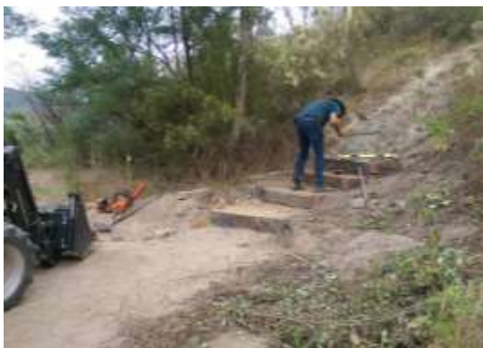
Will Ellis working hard on the new steps
